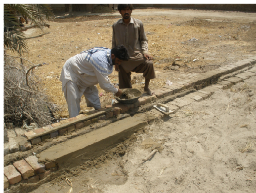
Construction of Sanitation Drain in Village Sahita, UC Jindodero, District Shikarpur
